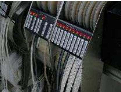
LED status display (green and red LED) and lane identification code.
