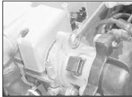
3.16 . . . then undo the retaining bolts . . .
