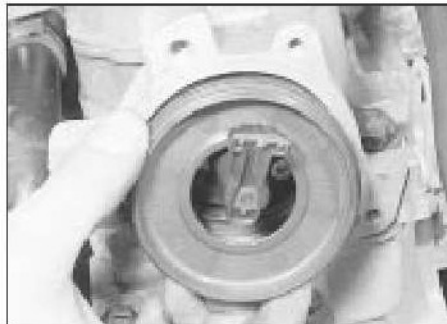
3.9 Extract the insulator
