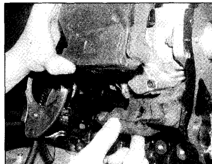
9.27 Refit the foam insulation pieces
