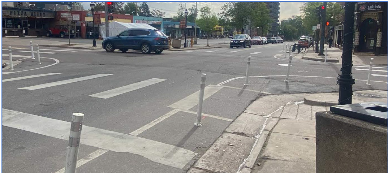
Figure 3: A rapid response countermeasure to install daylighting with flexible delineator posts in commercial area with heavy pedestrian volumes with the goal “to slow vehicles and shorten the crossing distance”
