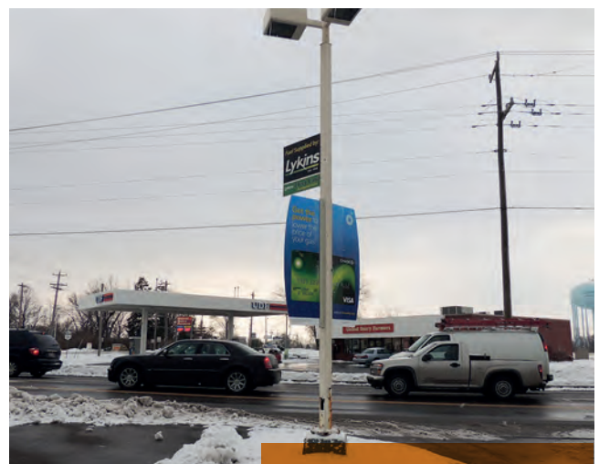
Figure 34: Permanent light pole with temporary sign components.
