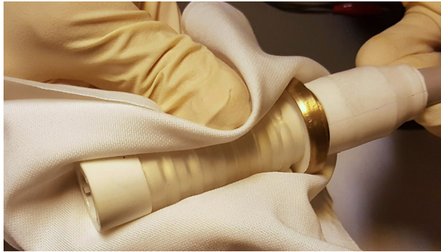
Figure 10 - Cleaning the cable connector
