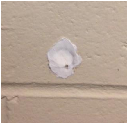
Hole patched with silicone RTV
