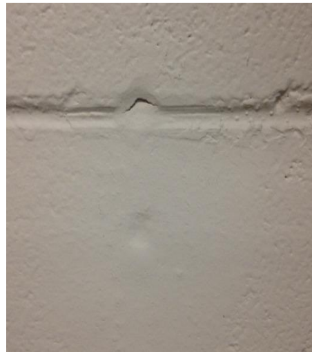
Holes patched with plaster compound
