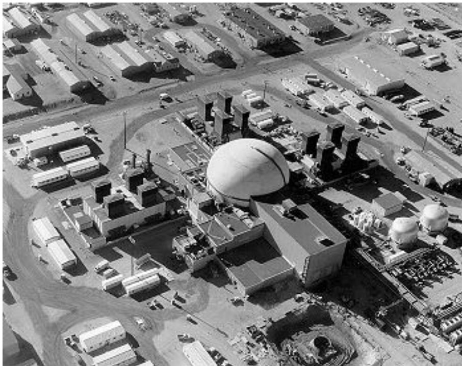
FIG. 2.68. Aerial view of the FFTF site, clearly showing the containment dome of the reactor and its three sets of four air-dump heat exchangers.
