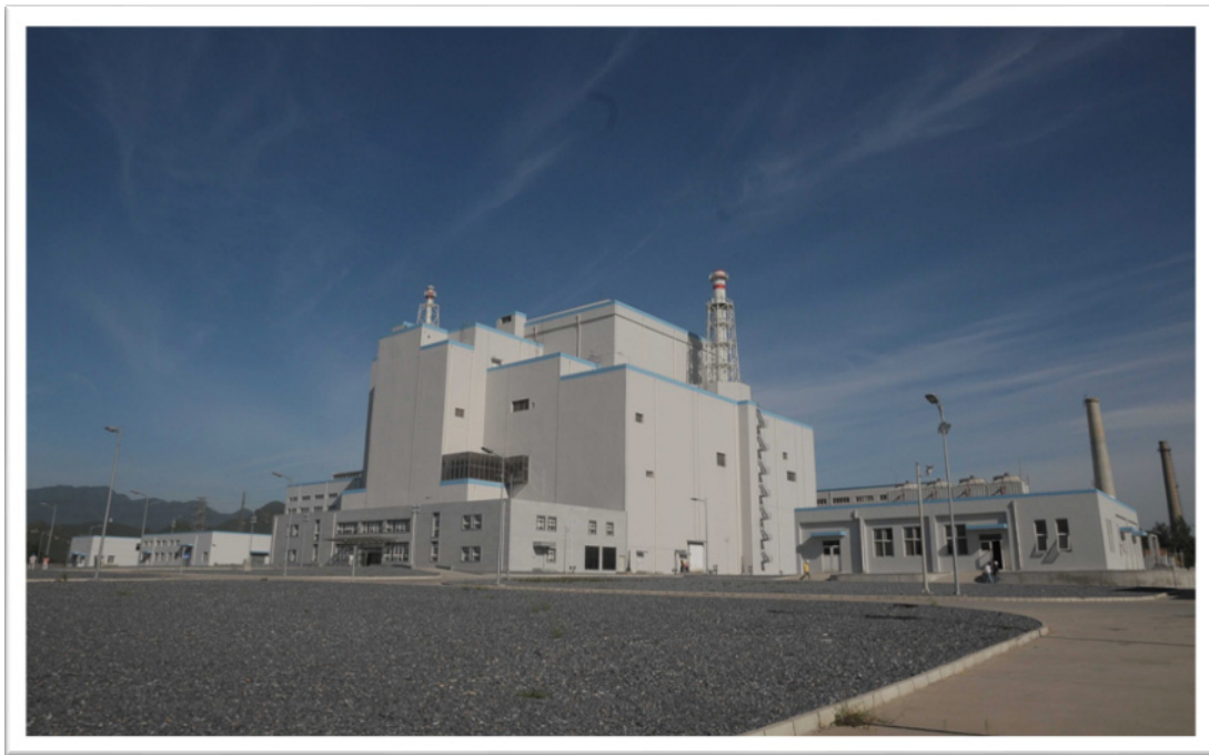
FIG. 3.6. CEFR reactor building.
