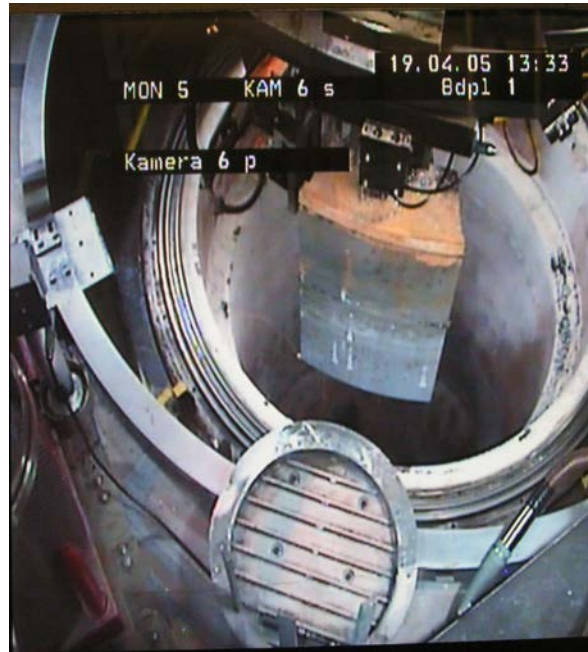
FIG. 2.52. Lifting reflector part from the reactor vessel.
