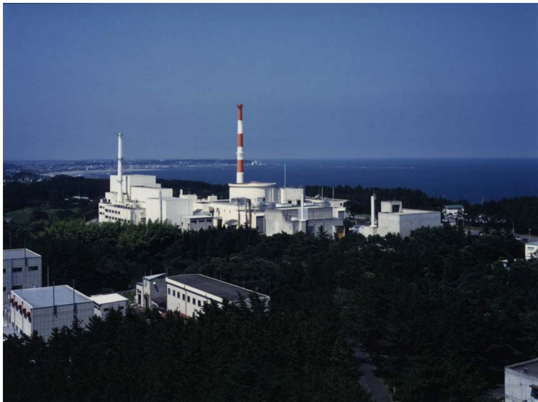
JOYO overall survey.
