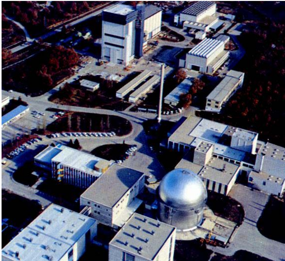
Rapsodie overall survey.
