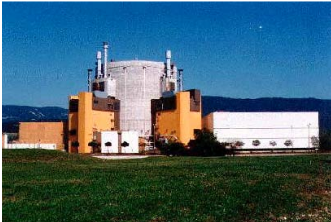
Super-Phénix 1 overall survey.
