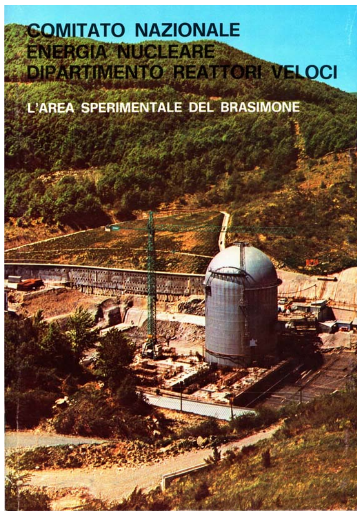
PEC reactor plant: the site of construction (1 of 2).
