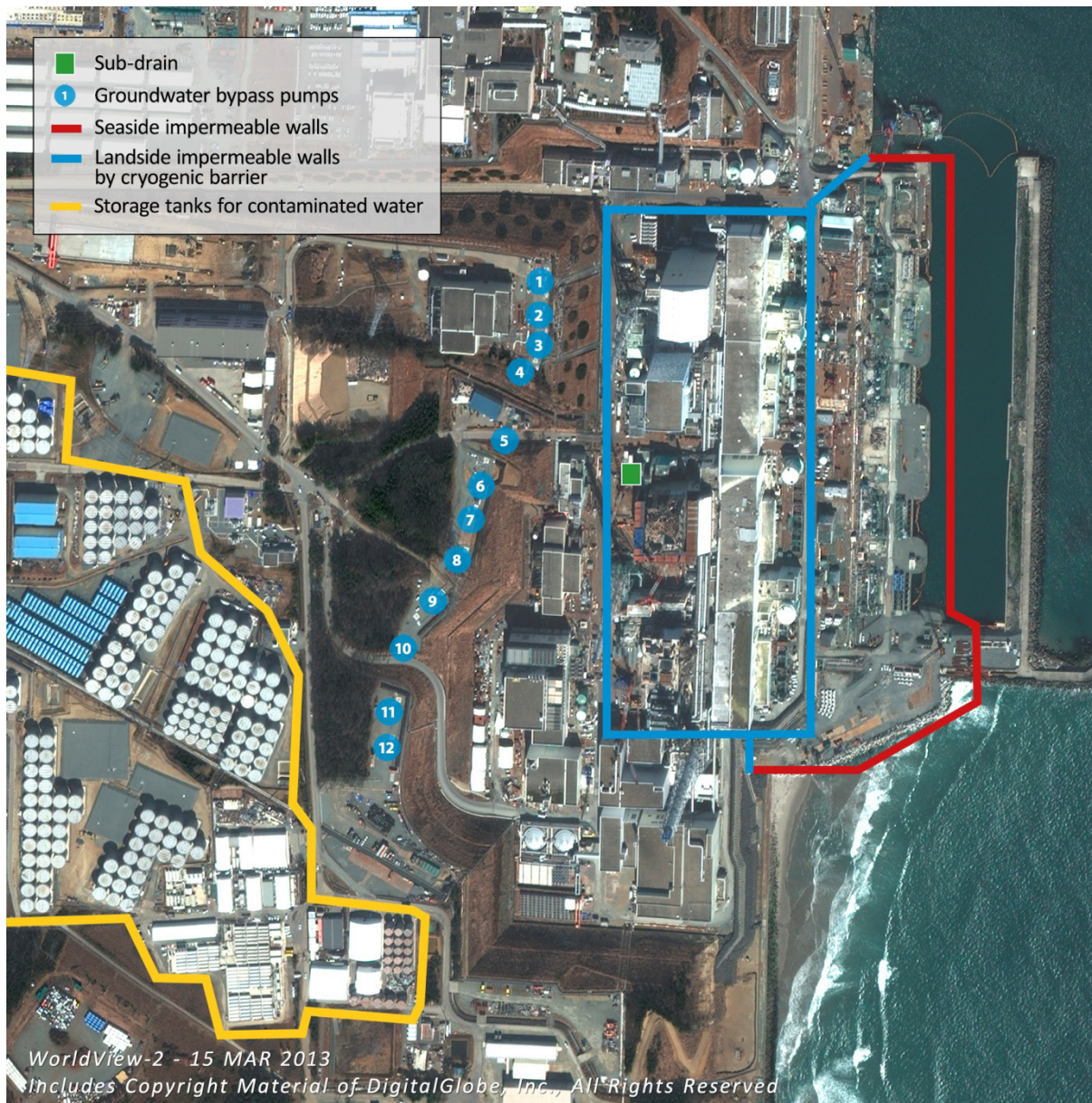
FIG. 5.5. Illustration of water management efforts. Storage tanks for contaminated water are shown on the left [286].
