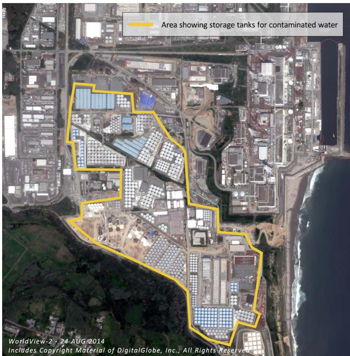
FIG. 5.8. Aerial view of the on-site area showing the water storage tanks [301].
