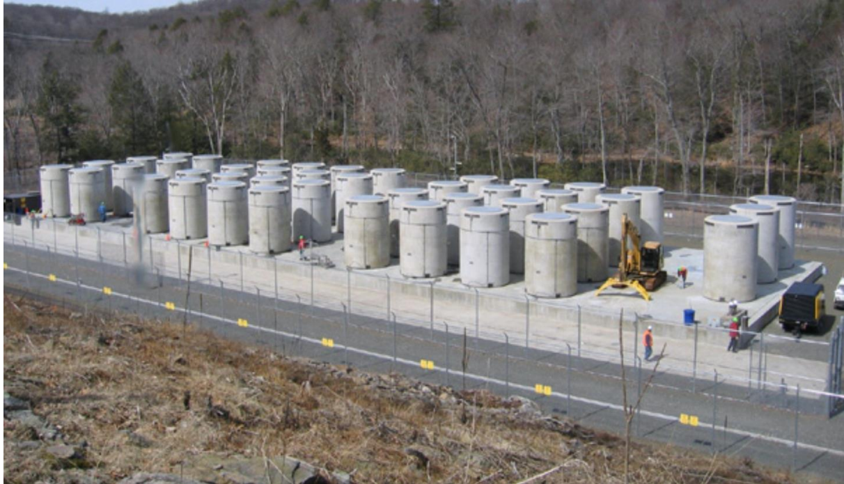
Fig 19: All the waste from a 450 MWe nuclear reactor for 28 years. If coal plant ash for the same energy was placed on this pad, it would be a column 2000 m high.
