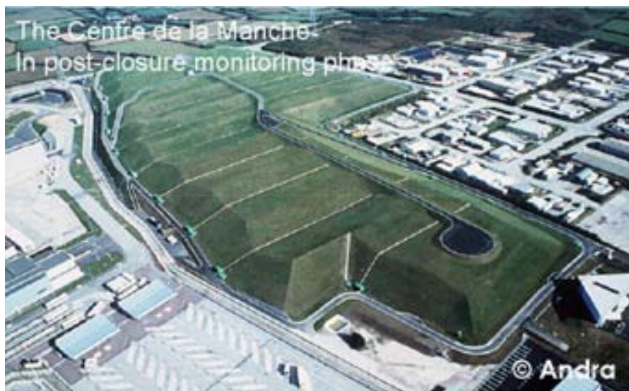
FIG. 16. Aerial view of the Centre de la Manche. A multilayer, non-permeable cover protects the waste disposal area (courtesy of ANDRA).
