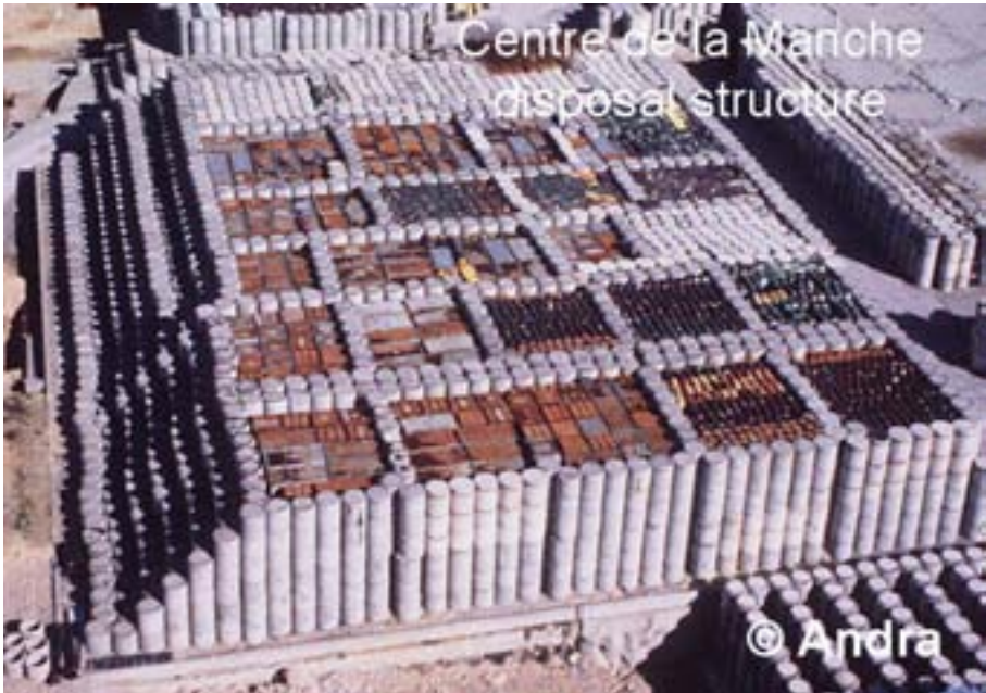
FIG. 15. Tumulus of concrete packages and metal boxes at the Centre de la Manche (courtesy of ANDRA).
