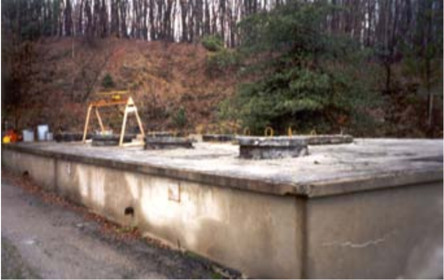
FIG. 11. Disposal vault for solid waste before improvement.
