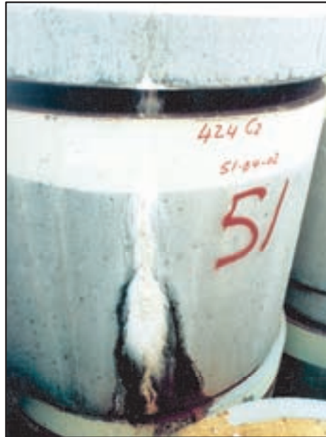
FIG. 28. Leachate from a cracked concrete container at Vaalputs.
