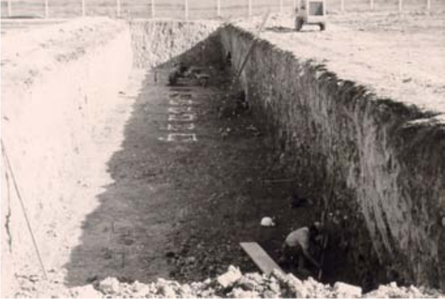
FIG. 14. Creation of the Centre de la Manche, 1969 (courtesy of ANDRA).
