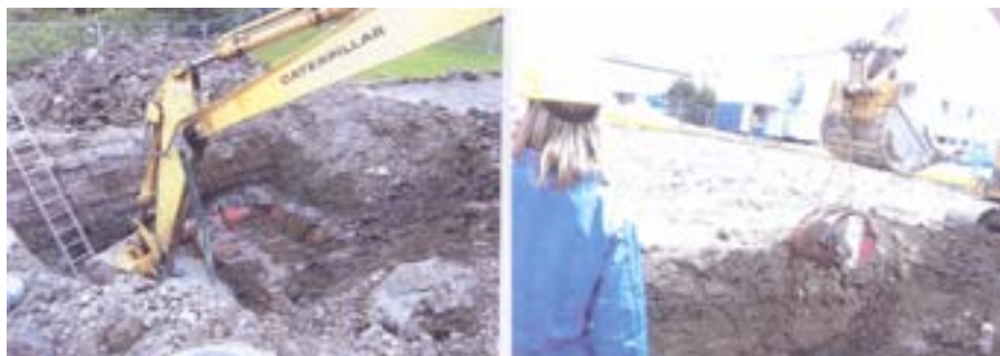
FIG. 23. Retrieval of waste drums at the Kjeller site.
