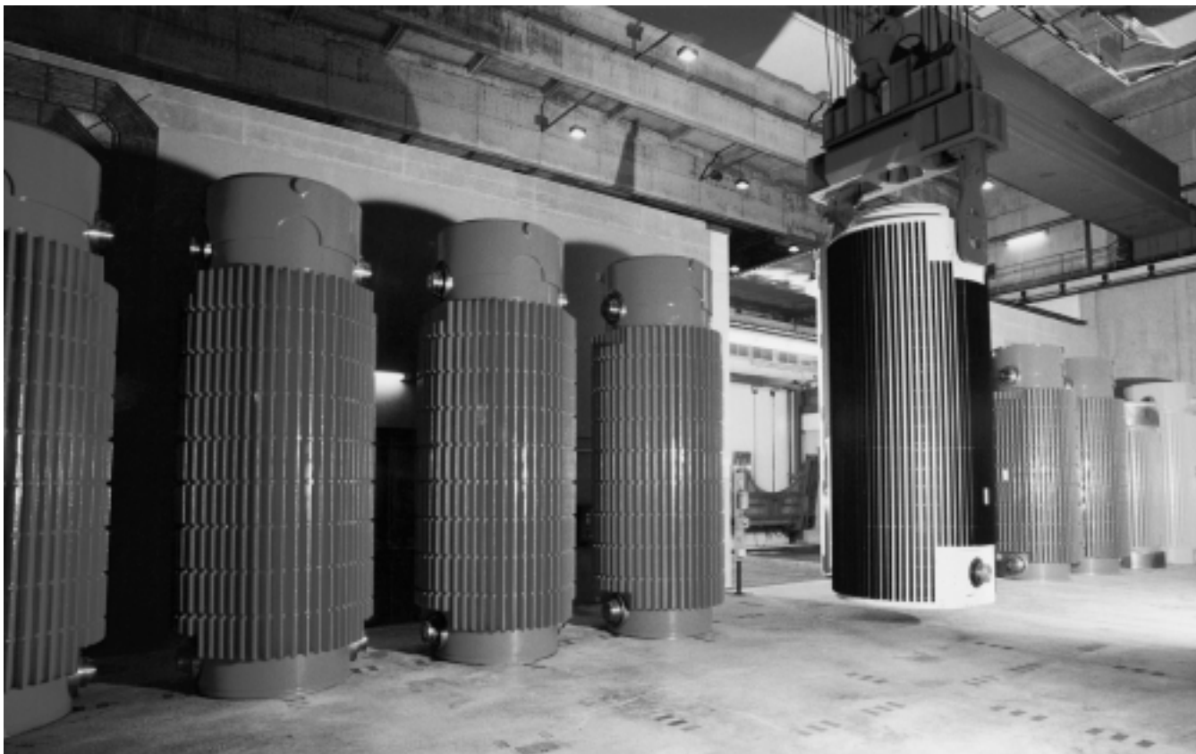
FIG. 22. Storage of spent fuel transport casks (Germany).
