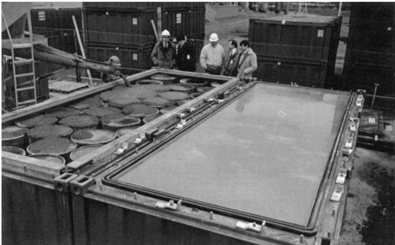
FIG. 9. Grouting of a container filled with LILW drums (UK).
