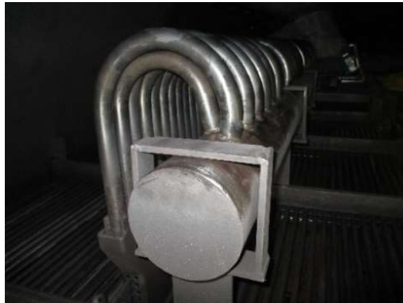
FIG. I-3. Feed water distribution piping from CEZ a.s., Dukovany NPP. Reproduced from Intranet CEZ a.s., Dukovany NPP with permission.
