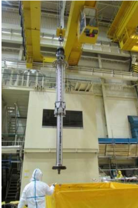
FIG. I-2. Decontamination equipment from CEZ a.s., Dukovany NPP. Reproduced from Intranet CEZ a.s., Dukovany NPP with permission.
