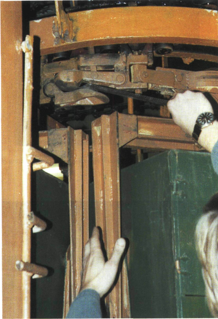
Photograph 6. Operator restoring conditions to normal with a metal rod.
