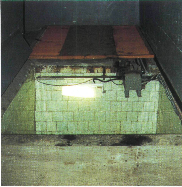
Photograph 9. Dry pit with moveable floor section at the maze entrance.
