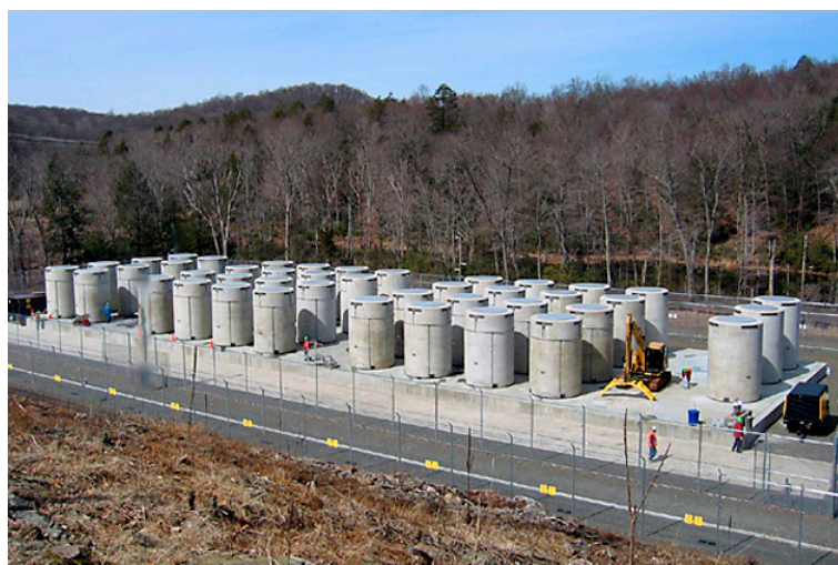
FIG. 20. View of a spent fuel dry storage facility.
