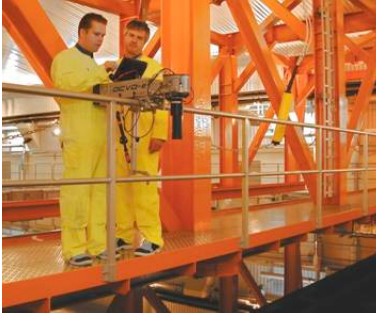
FIG. 19. DCVD in use in spent fuel wet storage.
