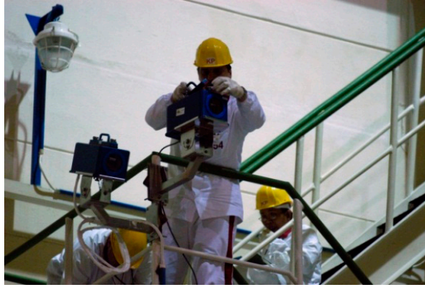
FIG. 10. Installation of a surveillance system.
