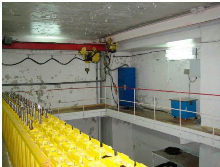
FIG. 11. Receipt and installation of IAEA equipment racks.
