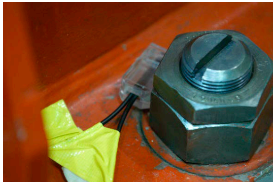
FIG. 9. Examples of seals that are used by the IAEA to maintain continuity of knowledge.
