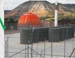
Operating ISF, José Cabrera NPP
