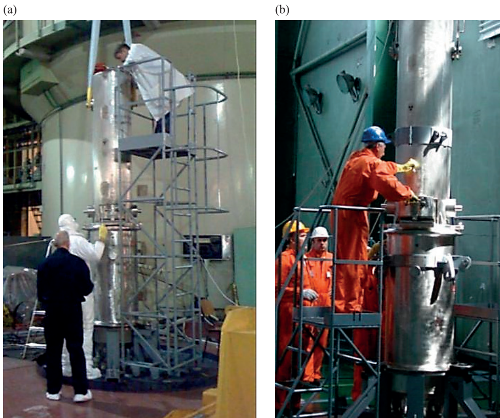
FIG. 33. Spent fuel assembly loading into the TUK-19 cask using transfer casks in Romania and Serbia.
