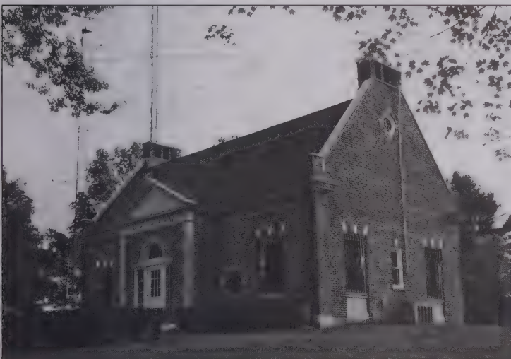
Figure 1.8 — This iconic brick building houses W1AW, the station operated by the ARRL in Newington, Connecticut, and known around the world. W1AW memorializes Hiram Percy Maxim, one of the founders of the ARRL. Visitors are welcome and often operate the station. [Rick Lindquist, WW1ME, photo]
