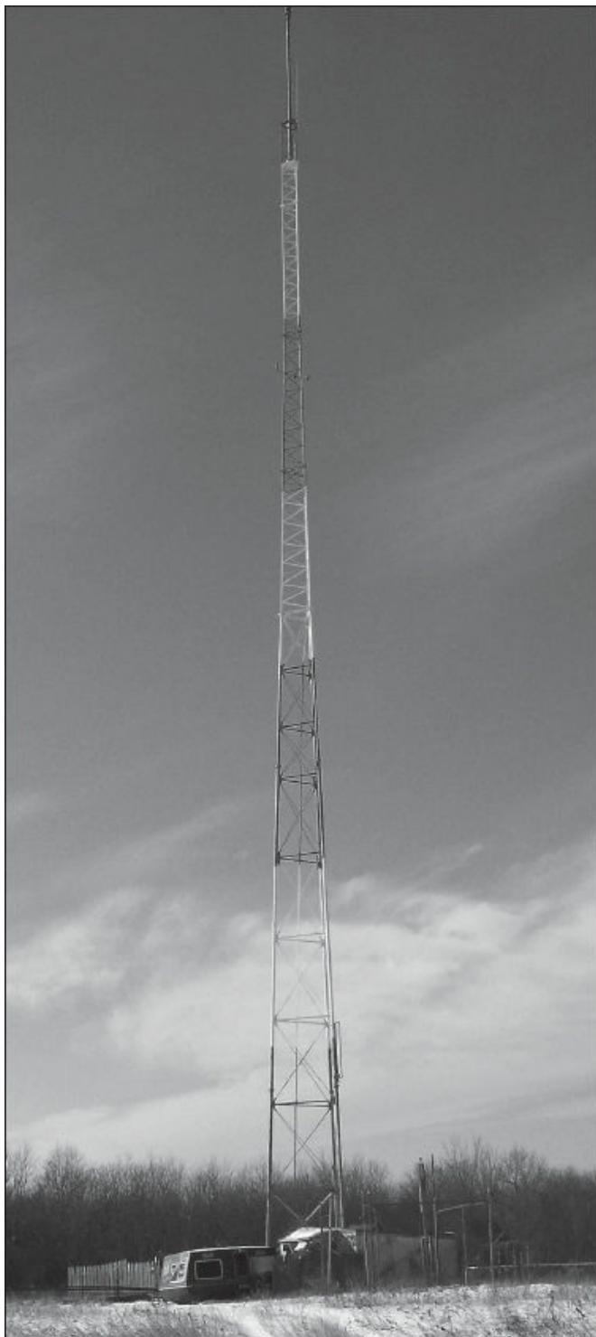
Figure 1.10 — Typical \frac{1}{4} wave AM broadcast vertical monopole antenna. The steel tower itself and the ground radial system comprise the antenna. AM broadcast antennas are usually located over the best conducting soil possible to enhance the desired ground wave as we will explore in depth in Chapter 7. Wet soil enhances ground conductivity significantly. [Richard B. Johnson, photo]
