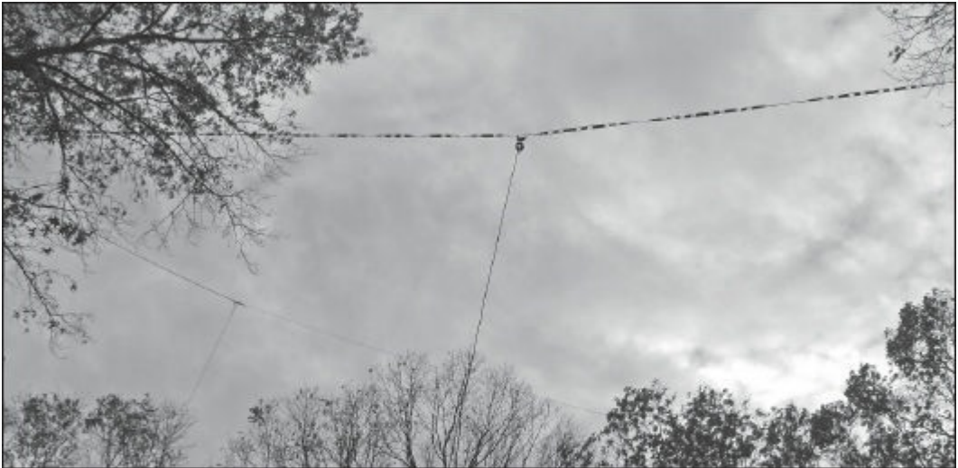
Figure 2.16 — Two much longer dipole antennas, one for 3.5 MHz (in the back-ground) and the other for 7 and 14 MHz. Notice that the dipole in the foreground uses “open wire” feed line for the radiating element, with one of the two conductors cut for 7 MHz and the other for 14 MHz. Functionally they are identical to the 950 MHz dipole in Figure 2.15 except for the wavelength of operation. [Joel Hallas, W1ZR, photo]
