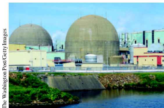
Figure 20.2.5 The North Anna nuclear power plant near Charlottesville, Virginia, which generates electric energy at the rate of 900 MW. At the same time, by design, it discards energy into the nearby river at the rate of 2100 MW. This plant and all others like it throw away more energy than they deliver in useful form. They are real counterparts of the ideal engine of Fig. 20.2.1.
